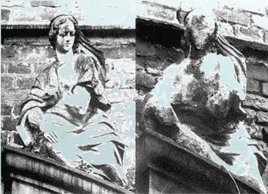
How acid rain affects stonework. The picture on the left was taken in 1908. The picture on the right was taken in 1968
